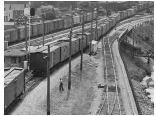
HISTORICAL PHOTO OF MEMONONEE VALLEY INDUSTRIAL CORRIDOR
